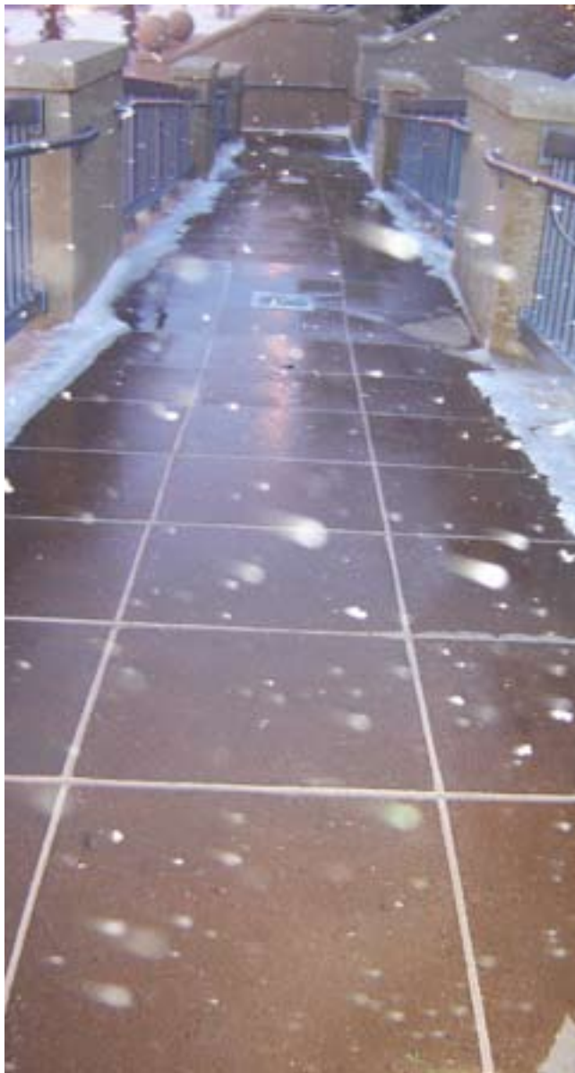
The pavers can reach 100°F when the ambient outdoor temperature is 0°F.
