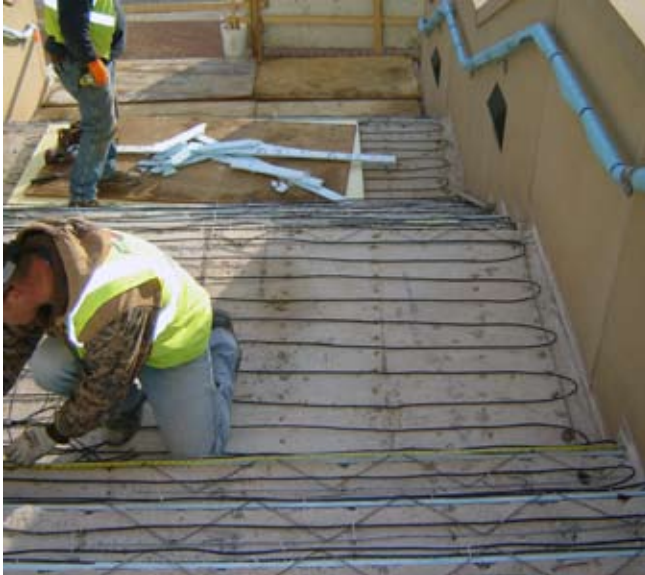
The M.I. snow melting cable assemblies are tied to rebar before the concrete is poured.
