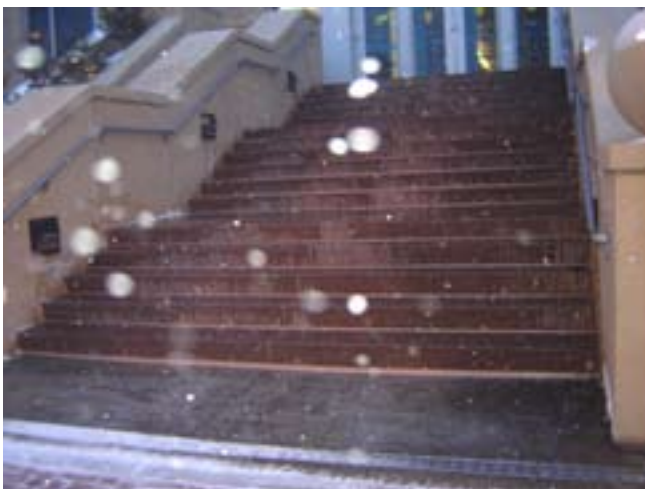
Snow melted stairs prevent accumulation and provide safe access during a storm.
