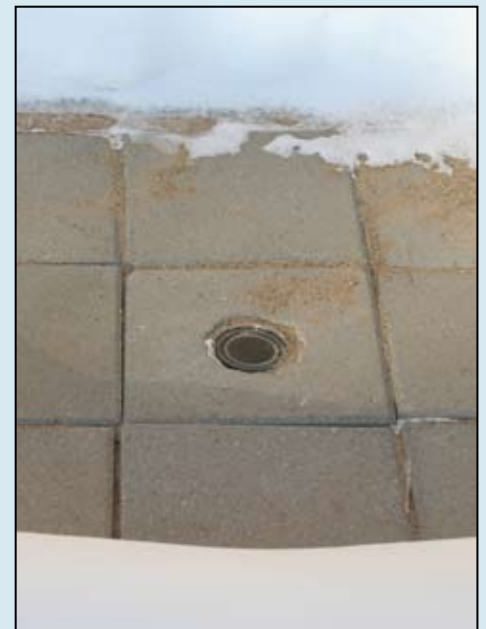
Snow Sensor Test Pad has melted the snow accumulation.
