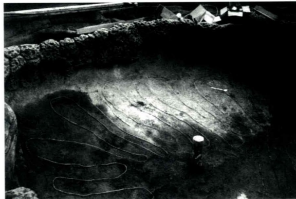
MI cable installed at the Cincinnati Zoo albino alligator exhibit
