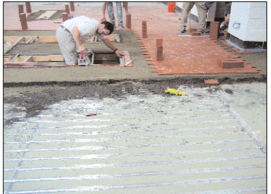
After the 2FW floor warming cable is laid and taped, German Klinker tiles are installed. These tiles are used in all BMW facilities, and they are installed by hand for precision. The tiles form an effective radiant surface for employees' comfort.
