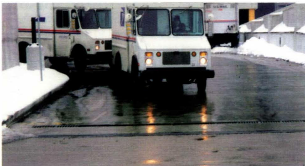
Designers of the new Main Post Office in Chicago knew that a snowmelt system would be the only practical method to keep ramps and driveways clear.
