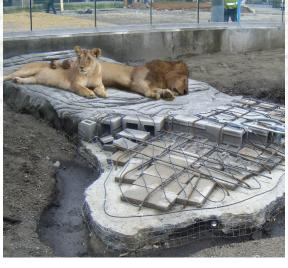
The two rocks were treated with seamless copper jacketed, single conductor M.I. cable covered with a high density polyethylene overjacket. Later, the skeletal structures with attached cables were solidified with gunite (cement, sand and water applied through a pressure hose) to create a rock-like surface. One rock is 133 square feet; the other is 144 square feet.
