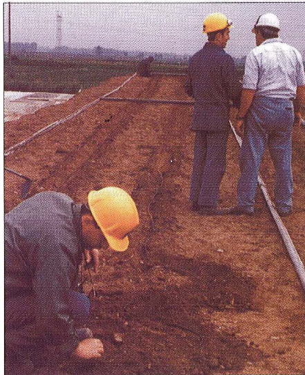
Workers laying out mineral insulated cable.
